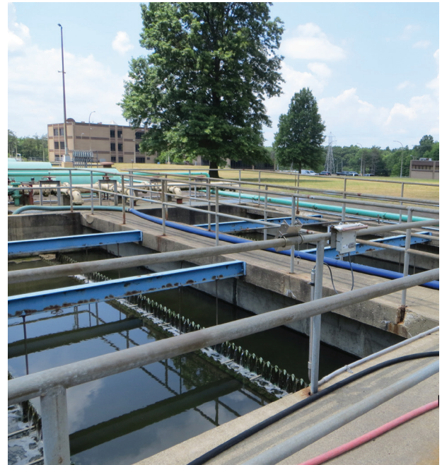
Meander Water Pollution Control Facility
